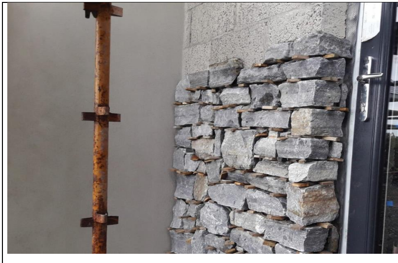
Figure 2 Filling of gaps between the stones with small stones and spacers
