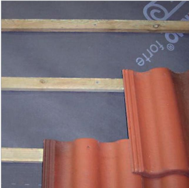
Permo<sup>®</sup> forte is an extremely strong 4-layer vapour permeable underlay with a built-in safety grid. It is suitable for all pitched roofs. Permo<sup>®</sup> forte should be laid in accordance with our installation details and BBA/IAB Certificates.
